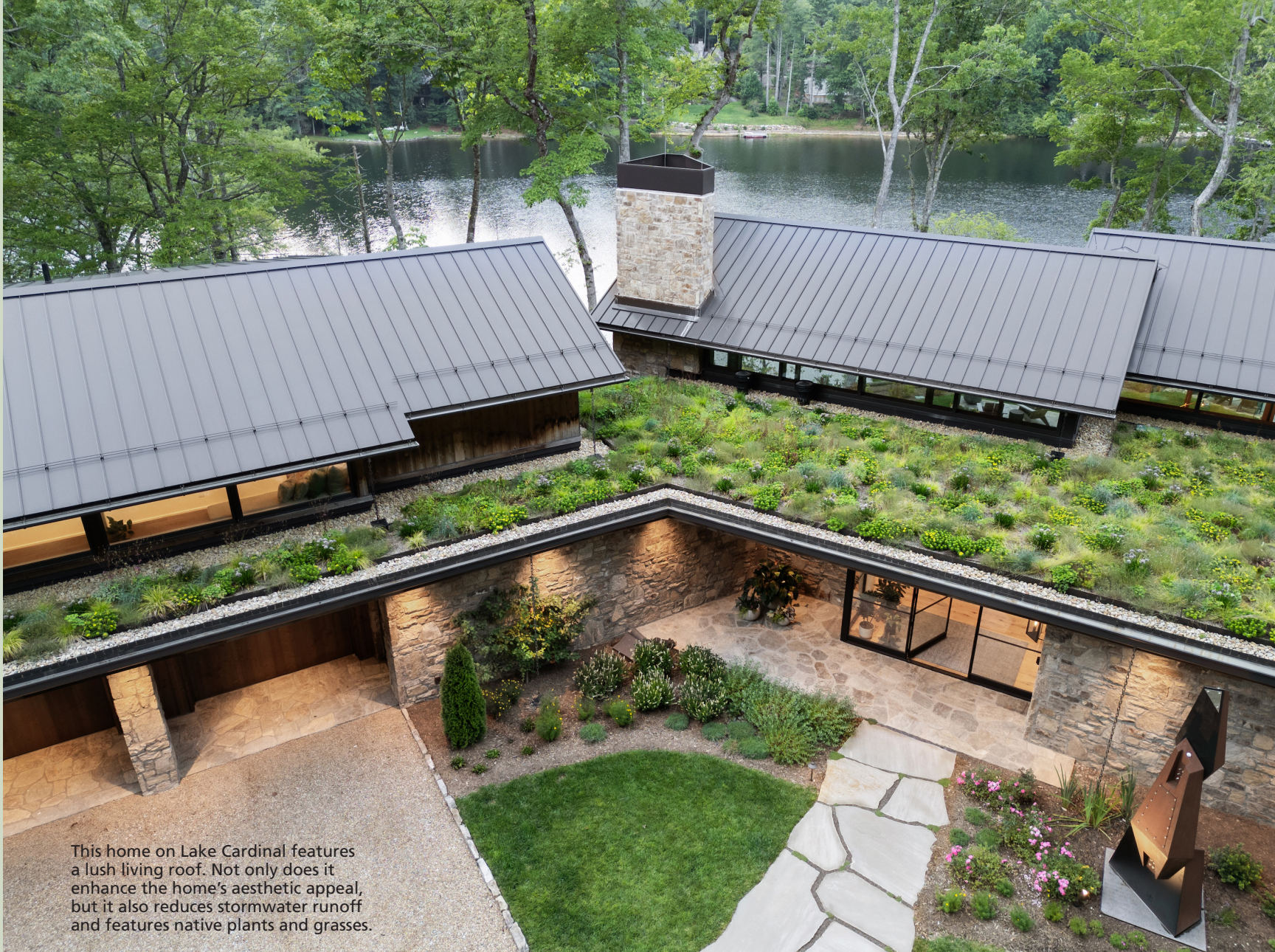
Patio pavers with large gaps and planted joints, while not technically pervious, allow runoff to infiltrate the root mat of plants. Vegetation absorbing some of the runoff and slowing down the rest helps lessen impact as water leaves the patio and can reduce the volume exiting the site.
